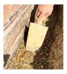
Dig out 250mm out from the wall, dig down 250mm allowing space for the pea shingle & possibly a land drain should invert levels allow.
