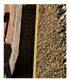
The Air Drain is 150mm wide & 200mm deep, it can be cut where need be, then we back fill with pea shingle to the face of the air drain.
